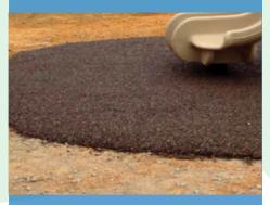
The rolled edge application is the most commonly used method. The edge of the surfacing will die into a trench around the sub base. After the surfacing is installed the dirt from the trench is used to backfill against the surfacing.
