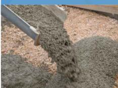
Concrete is also an acceptable sub base. It can be the most expensive depending on your location and square foot area. The concrete thickness should be at least 4" and no less. Be aware that if your area is in a courtyard or difficult to access, you will need a pump truck.
